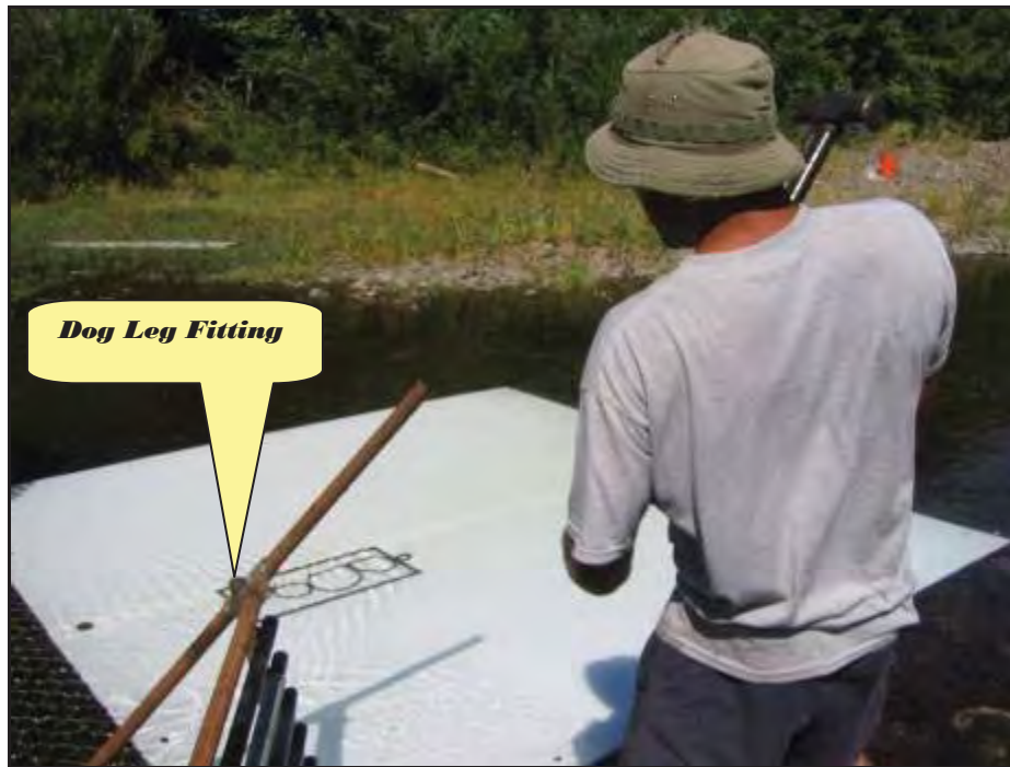
Figure 9. Construction of the weir. Dogleg fittings were bolted to the uprights and the “weir arm” slides through the fitting. This was pounded into the stream bottom at a 45 degree angle downstream.
