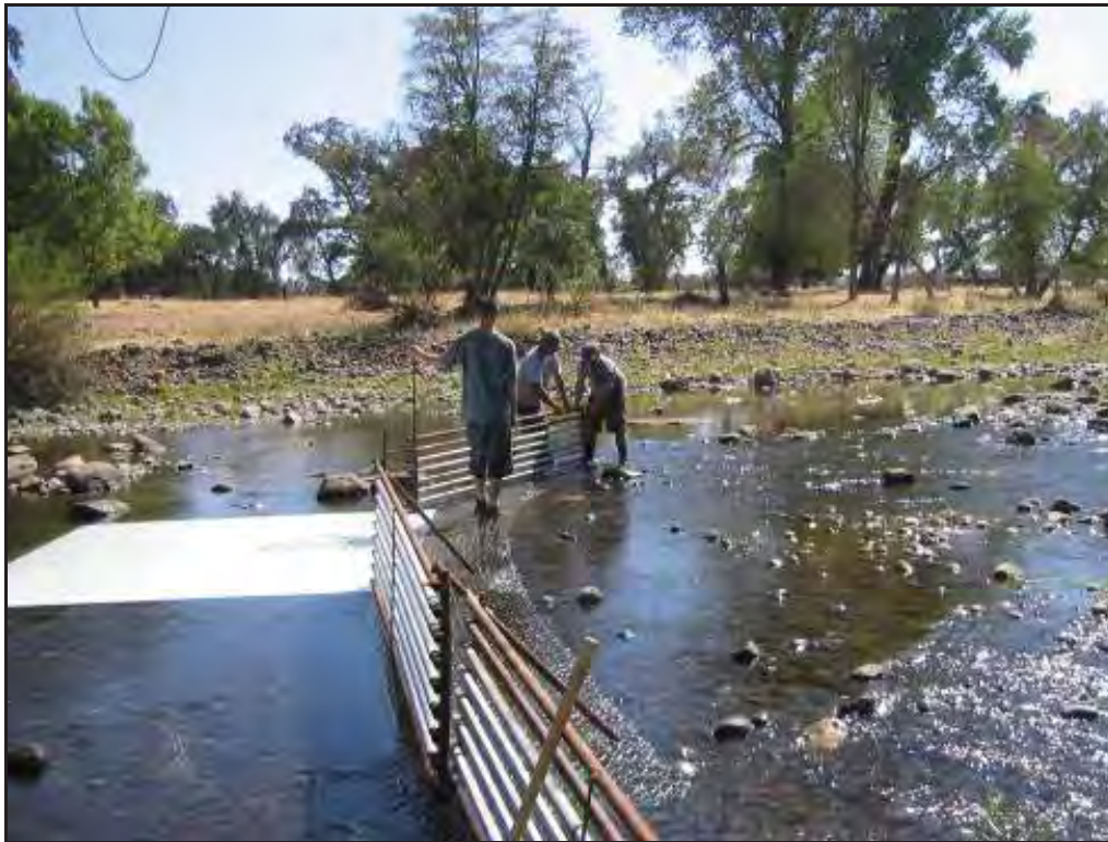
Figure 10. Construction of a weir included white high density polyethylene (HDPE) sheets staked to the creek bottom to make the observation of passing salmon easier.
