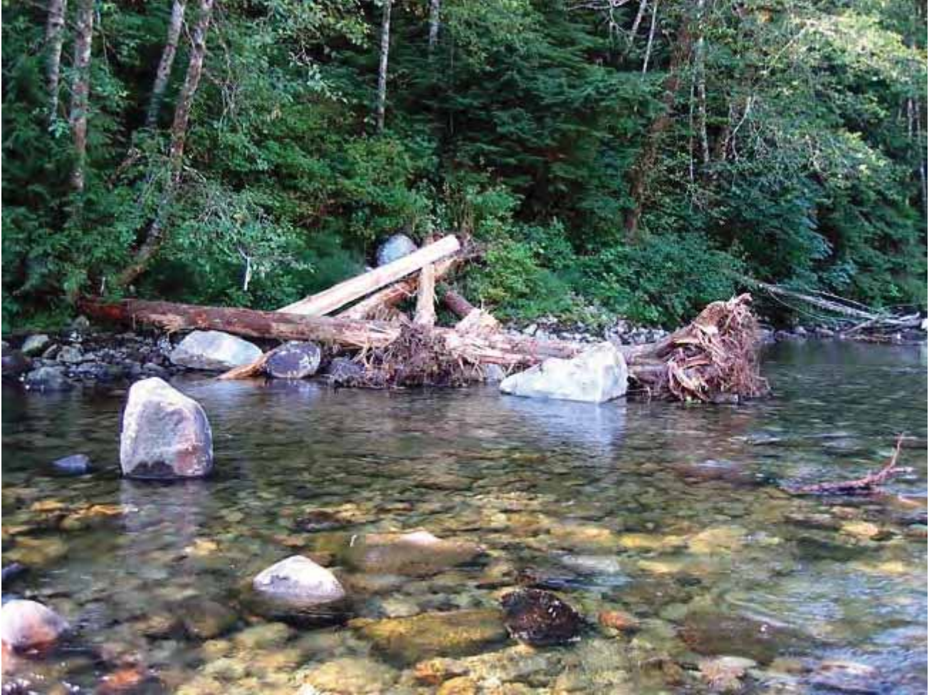
FIGURE 2 SPUR CONSTRUCTED FROM WOODY DEBRIS
