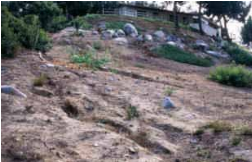
TOP: The downslope area adjacent to this residence has been denuded of all vegetation and is eroding. Meanwhile, fire hazards including a wooden fence and pine trees remain next to the house. • BOTTOM: Typical of many new developments in wild areas of Southern California, these houses were built too close to each other, and are surrounded by flammable trees. Their risk for damage from a wildfire is high. Photographs by R. Halsey.
